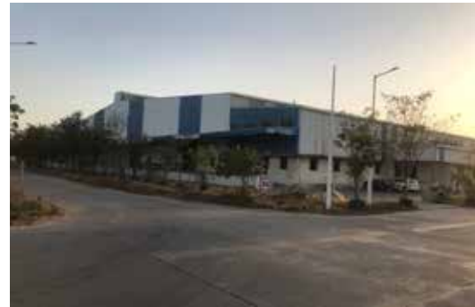
Filament Winding Shed
