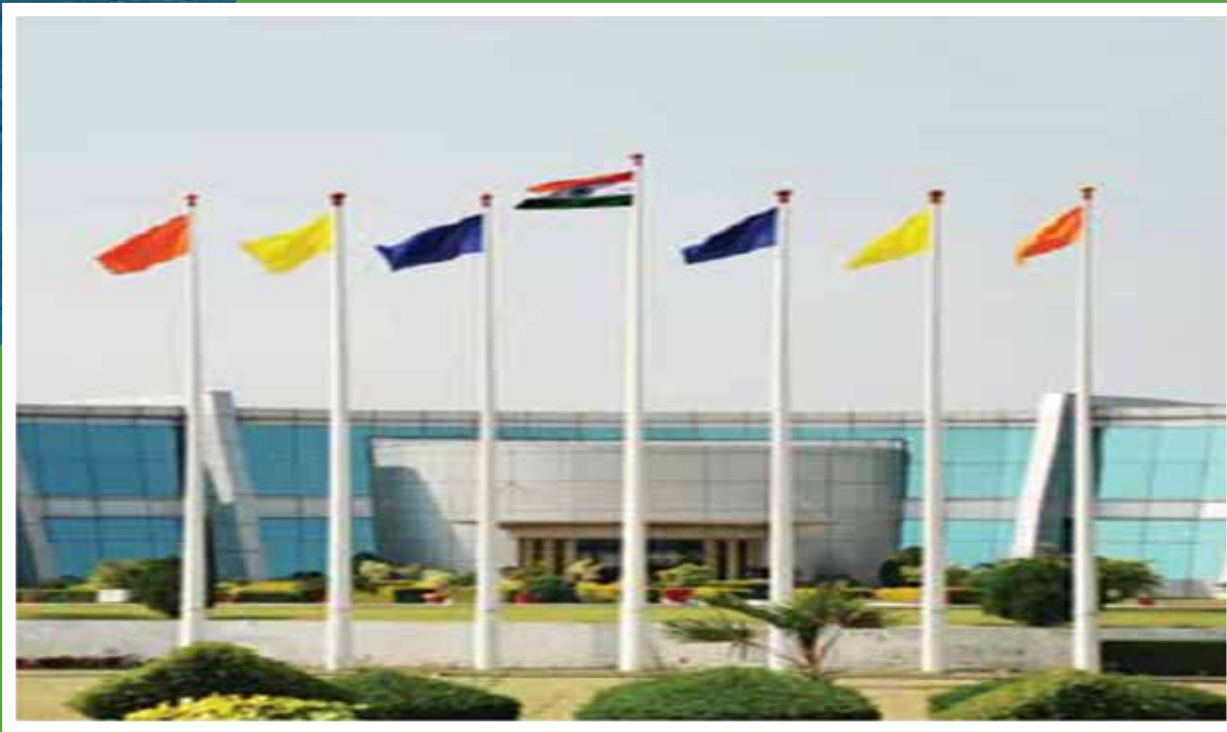
Reliance Composite Solutions – Vadodara, Gujarat
